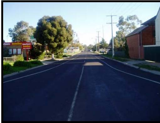
Photograph 4: Burns Street - View to South from Tuaggra Street
