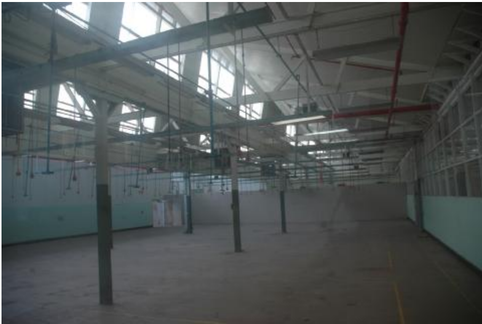
Photo 6 View of interior showing saw toothed roof and trusses.
