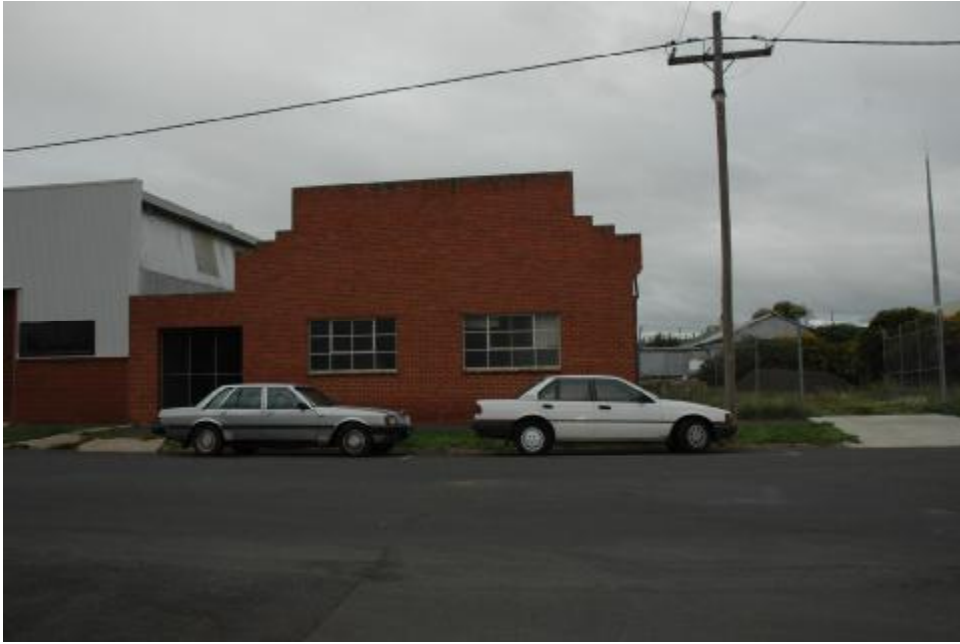
Photo 3 Possible early Boiler House
