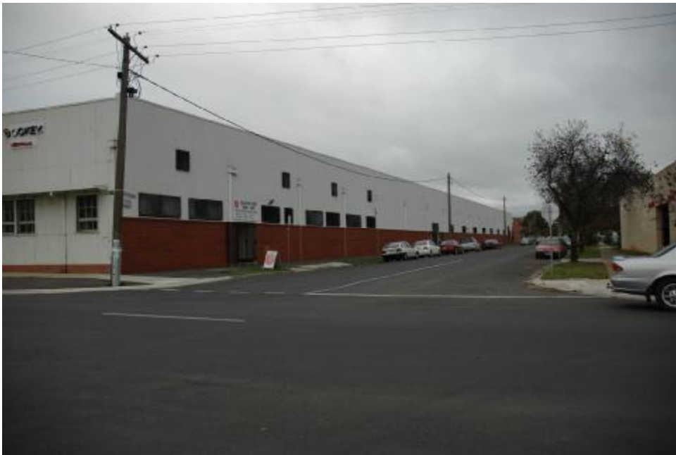
Photo 2 Burke Street Frontage
